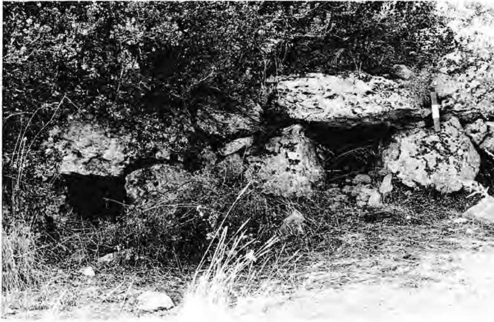
Fig. 21. Mycenaean road. Culverts on Kondovouni.
