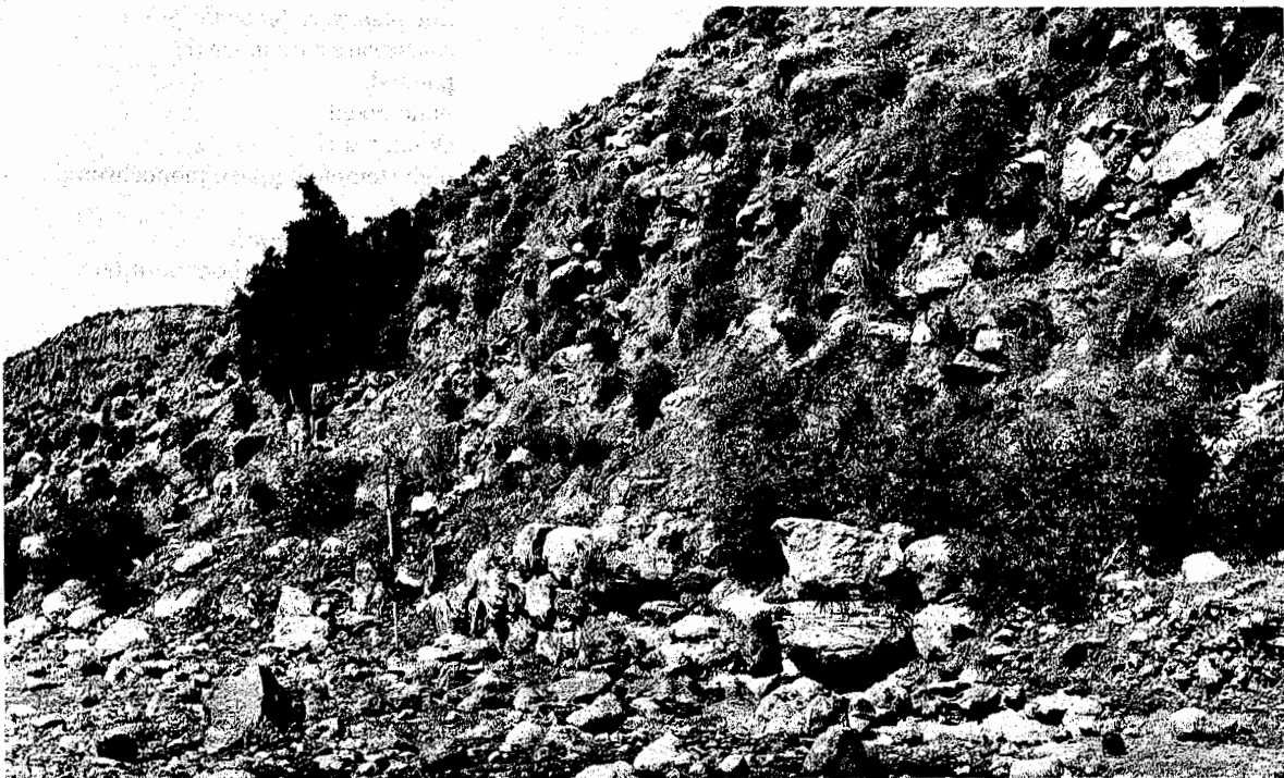
Fig. 10. Part of the east face of the Mycenaean dam. The dam was ca. 10 m high and protected by Mycenaean walls still visible below the tree and in the center of the photograph. (Courtesy Deutsches Archäologisches Institut, Athens, neg. TIR 68/326)
