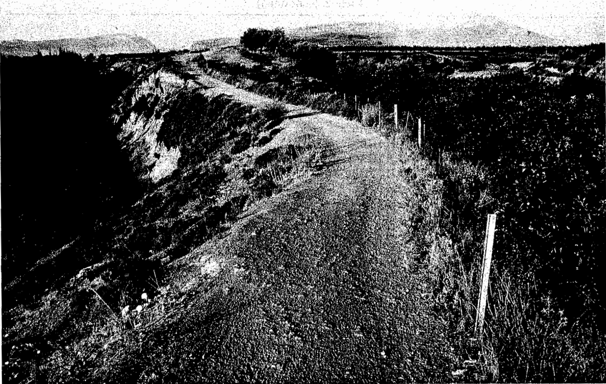
Fig. 9. Crown of the Mycenaean dam east of Nea Tiryns. The stream originally ran from the lower left to the upper right in the photograph. Since the diversion was carried out, the stream has run from the lower left through an artificial canal to the upper left.
