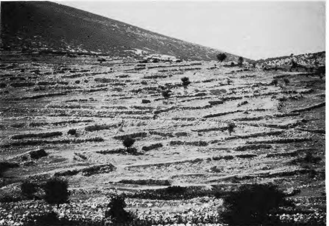
Figure 12.10 These terraces in the Limnes uplands belong to the second generation of terrace construction. They have been erected during the last 200 years and are still maintained today.
